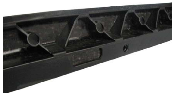
Fig. 2 Detail of the nylon composite sheet reinforcement for the lower beam
